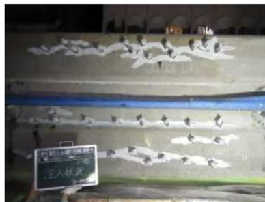
軌道桁(PC)のひび割れ補修
