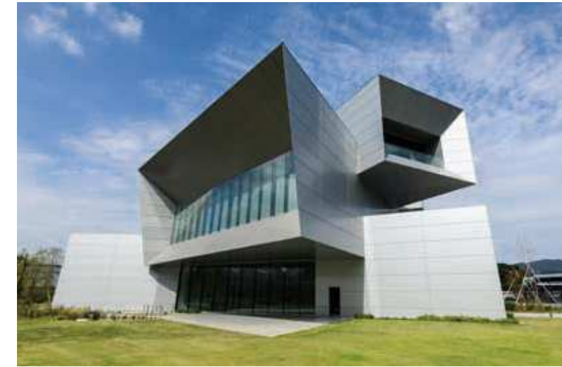
80 YASKAWA Innovation Center Address: 2-1, Kurosakishiroishi, Yahatanishi-ku Built in 2015 Blueprint: Mitsubishi Jisho Sekkei Inc. Photo credit: YASKAWA Electric Corporation
