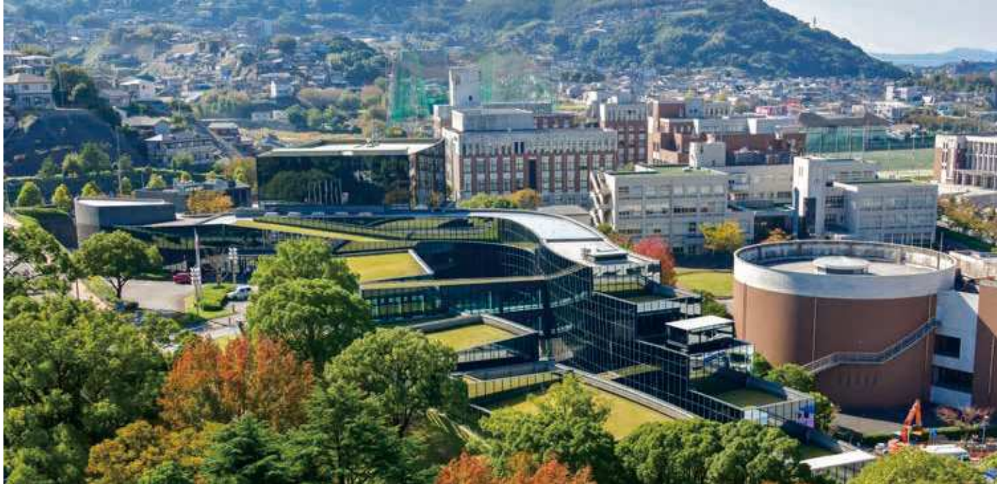
76 International Village Center Address: 1-1, Hirano, Yahatahigashi-ku Built in 1993 Blueprint: Ishii, Sum design JV
