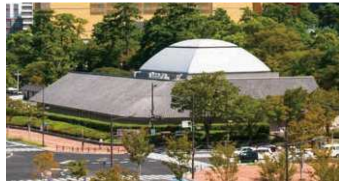
71 Matsumoto Seicho Memorial Museum Address: 2-3, Jonai, Kokurakita-ku Built in 1998 Blueprint: Tadanaga Miyamoto Architect & Associates
