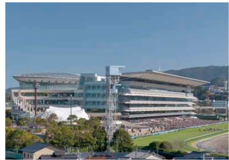
68 Kokura Horse Racing Track Address: 4-5-1, Kitagata, Kokuraminami-ku Built in 1999 Blueprint: JRA Facilities Co. Ltd. / Tohata Architects & Engineers
