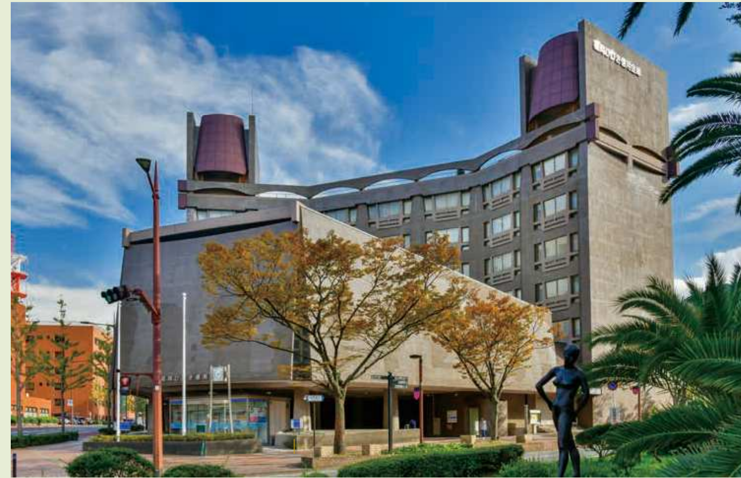
60 Fukuoka Hibiki Shinkin Bank Headquarters (Former Kitakyushu Yahata Shinkin Bank) Address: 2-8-1, Ogura, Yahatahigashi-ku Built in 1971 Blueprint: Murano Togo
