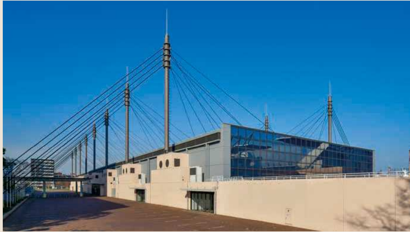
58 West Japan General Exhibition Center Address: 3-7-1, Asano, Kokurakita-ku Built in 1977 Blueprint: Arata Isozaki & Associates
