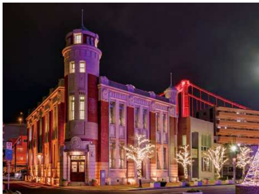
28 Former Furukawa Mining, Wakamatsu building Address: 1-11-18, Honmachi, Wakamatsu-ku Built in 1919 Blueprint: unknown
