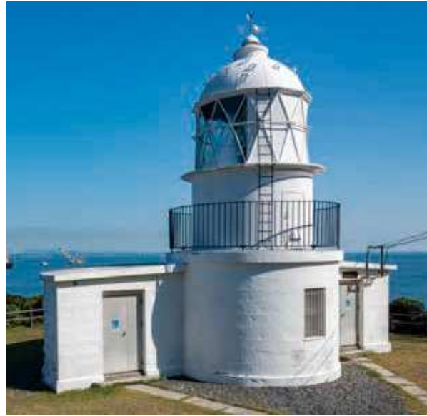
24 Hesaki Lighthouse Address: Oaza Shiranoe, Moji-ku Built in 1872 Blueprint: Richard Henry Brunton
