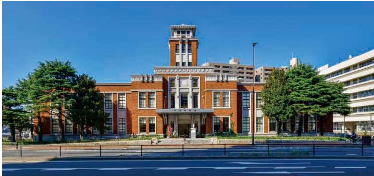
39 Tobata Public Library (Former Tobata City Hall) Address: 1-1-1, Shin-ike, Tobata-ku | Renovation 2014 | Blueprint: Shigeru Aoki Architect & Associates Address: Same as above | Built in 1933 | Blueprint: Fukuoka Prefecture Repair Division
