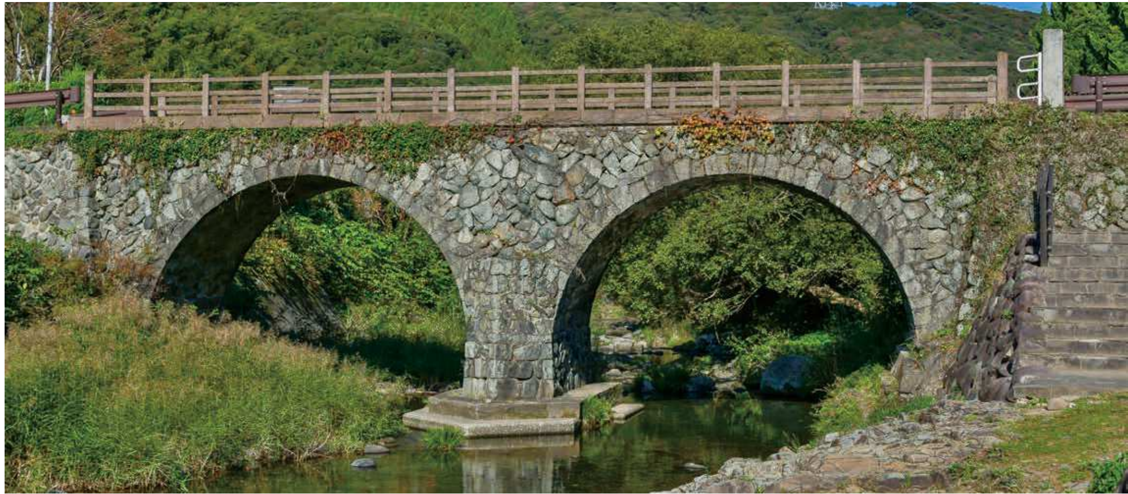
38 Haruyoshi Megane Bridge | Address: 397-7, Haruyoshi, Kokuraminami-ku | Built in 1919 | Blueprint: unknown
