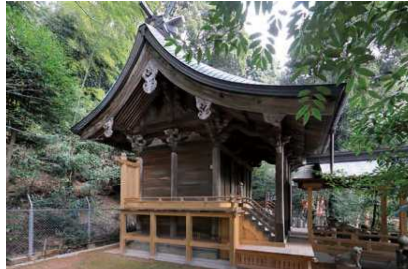
3 Kamo-hachiman Shrine main hall Address: 5-6-10, Gamo, Kokuraminami-ku Built in 1763 Blueprint: unknown
