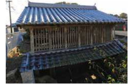
8 Jime-no-karato (sluice) Address: 3-12, Kusubashinishi, Yahatanishi-ku Built in 1804 Blueprint: unknown
